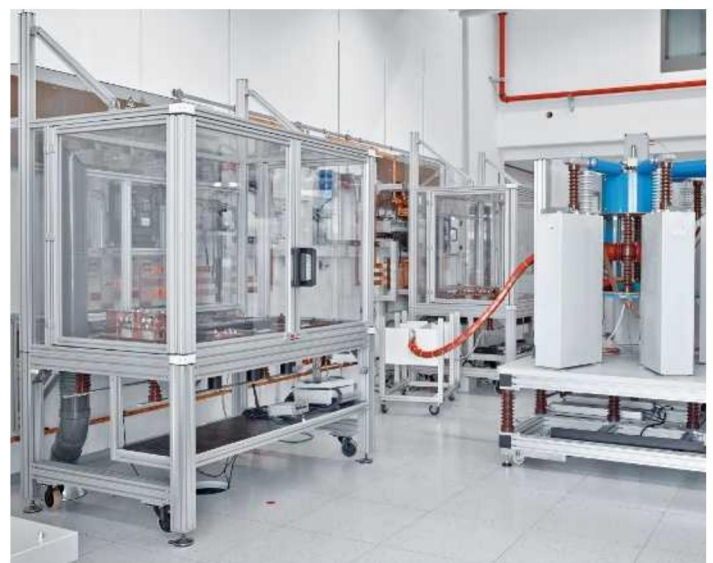
Fig. 25: Testing stations of the high-current testing system
